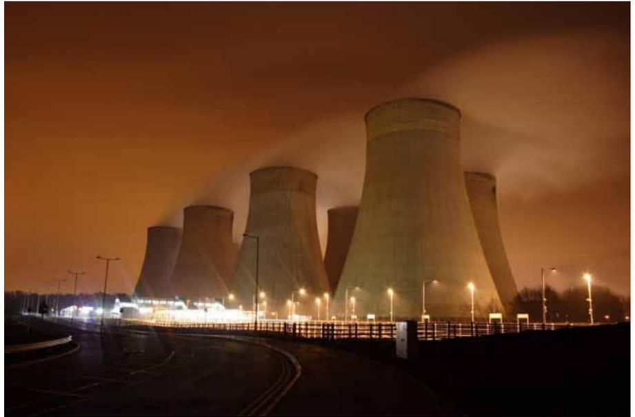
Figure 1. Natural Draft Wet Cooling Towers
