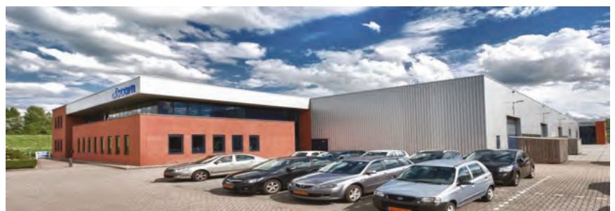
Figure 2. Discom B.V. headquarters in The Netherlands
